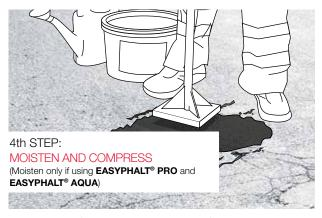
**EASYPHALT® PRO** and **EASYPHALT® AQUA** soak with water (about 5 litres of water per 25 kg bucket). Compress all EASYPHALT® with a roller, vibratory plate or hand tamper. The surface can be approved for traffic immediately after installation.
